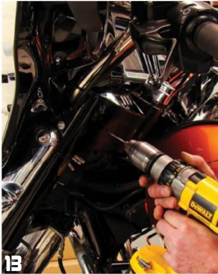
13 First, drill a pilot hole with a 1/8" drill bit.
