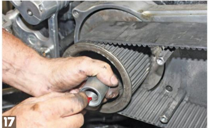
17 Now we come to the point in the installation that caused the original failure. The primary drive manufacture's tech said to put some blue or red Loctite on the insert nut to keep it from backing off.
